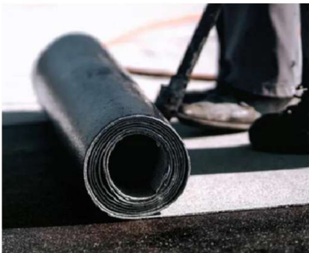
Bituminous Membrane Installation
